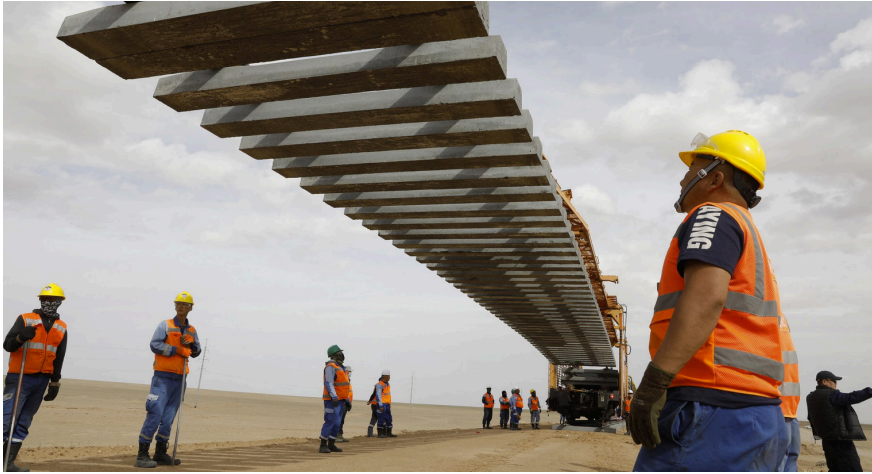
Fig. 7 Building the Tavan Tolgoi - Züün Bayan railway, Mongolia 2019 © 24 tsag.mn
