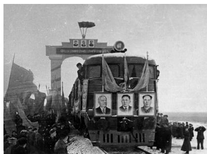
Fig. 3b Building the Ulaanbaatar-Zamyn Uud Road named Friendship, 1954 © Mongolian State Archive
